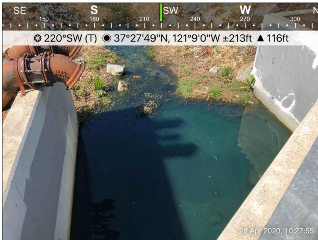
Photo 6: Detail of Salado Creek culvert at Sperry Avenue, view south.
