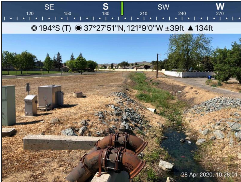
Photo 7: Overview of Salado Creek segment from the culvert at Sperry Avenue, view south.
