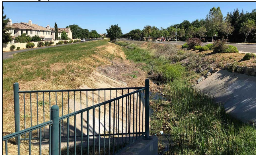
Overview of Salado Creek segment from the culvert at Sperry Avenue, view north.
