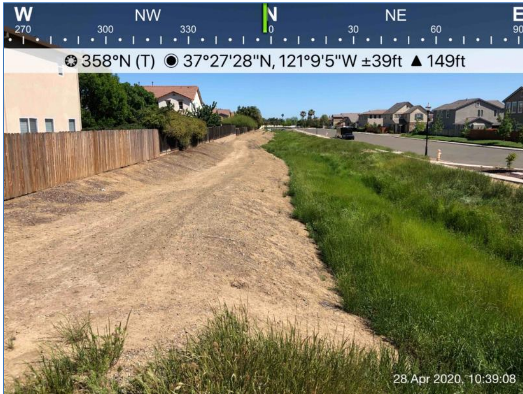
Photo 3: Overview from southern boundary of the APE (Sweet Briar Drive), view north.
